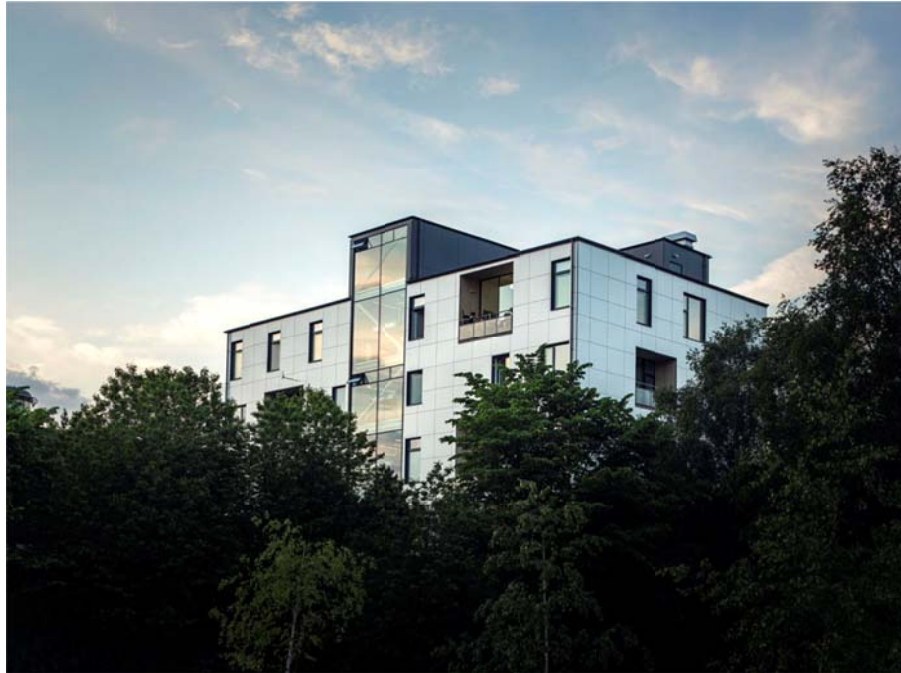
Figure 2: Outside view of HSB Living Lab at Johanneberg district, Gothenburg
