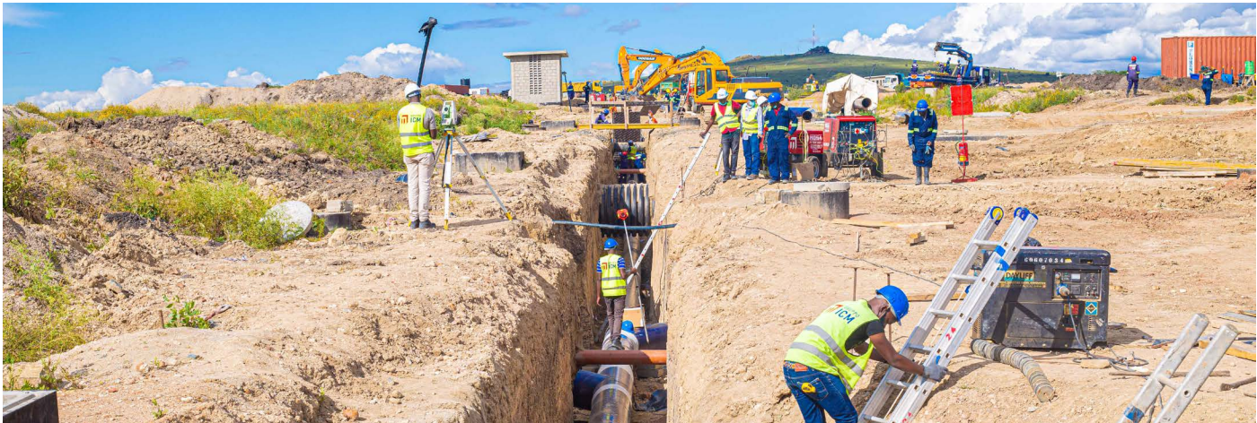
The ongoing horizontal infrastructure development at Konza Technopolis.
