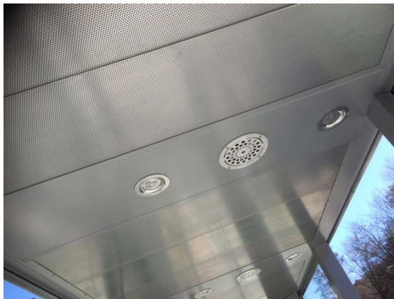
Figure 6 Detail (ceiling) of sound-proofed bus shelter
