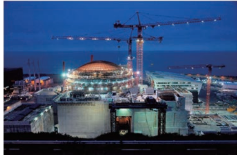
EPR nuclear reactor under construction Source EDF – Morin Alexis
